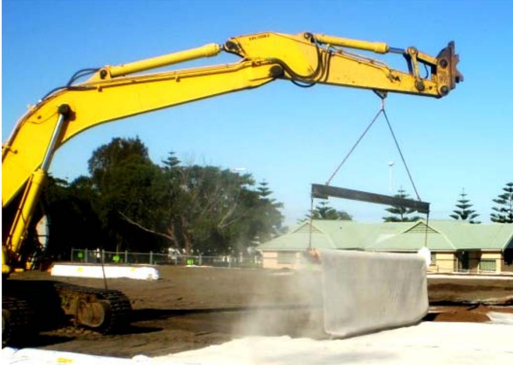
**FIGURE 1 – LOSS OF POWDERED BENTONITE DURING GCL DEPLOYMENT**
